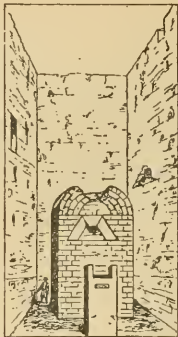
FIG. 22. Building in Campbell's Tomb. From Vyse.
