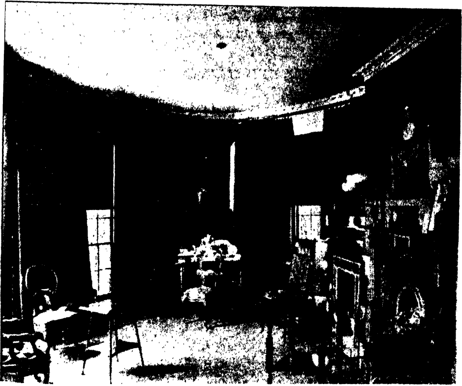
Interior, 73 Dana Street, Cambridge.
