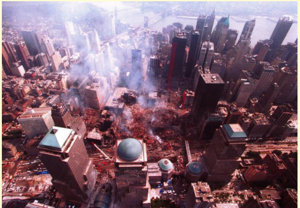
The photo above shows the rubble of the World Trade Center Complex after the attacks and collapses of World Trade 1, 2, and 7.
