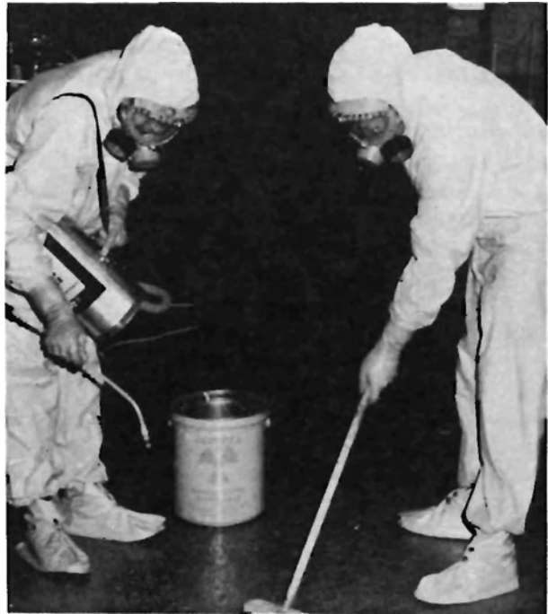
A professional decontamination team at work. Although workers are taking elaborate pains to see that no radioactive material touches them, the fundamental activity is no more complex than scrubbing the floor. (Photograph courtesy of Nuclear Associates, Inc., 100 Voice Road, Carle Place, New York 11514.)
