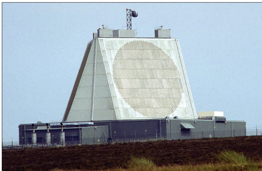
The Solid State Phased Array Radar (SSPAR) at RAF Fylingdales, UK. (Image: wikipedia.org)
