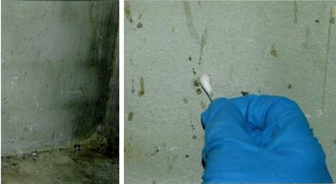
In a back corner of the meter room, next to the axe and sledgehammer, we found a rain of stains that rose up the wall. Right, a close up of some of the droplets, which field-tested positive for blood. Photos courtesy Jan Johnson
