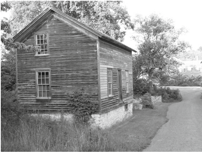
Fig. 5.9 A middle-class house on Sheldon Avenue. Note the foundations for another house to the right , and the extant hotel in the background
