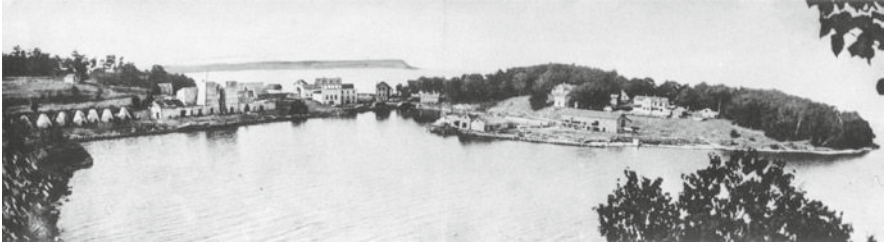
Fig. 1.5 View of Fayette townsite, circa 1907. Snail Shell Harbor is in the foreground. Notable features from left to right are several charcoal kilns, furnace complex, administrative and commercial buildings, and a knoll that housed upper and middle-class employees. Photo provided courtesy of the Michigan Historical Museum
