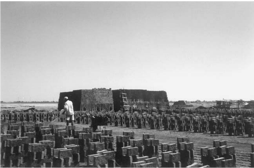
Plates 9 and 10. Foreground: Unfired bricks stacked to dry. Background: A brick kiln.
