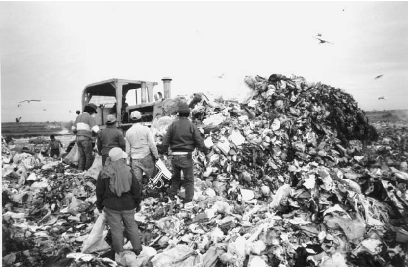
Plates 15 and 16. Bulldozer flattening and moving forward the garbage.
