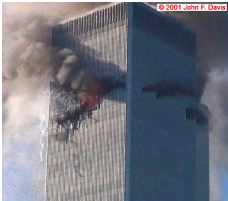
Figure 2–2. Aircraft entry hole on the north side of WTC 1, photographed 30 s after impact.
