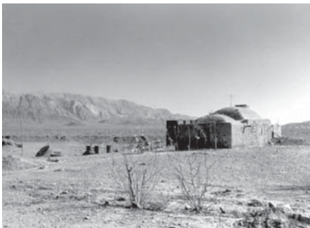
The police office on the outskirts of town
