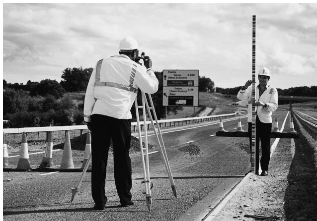
Figure 2 Surveying With Optical Level and Rod
