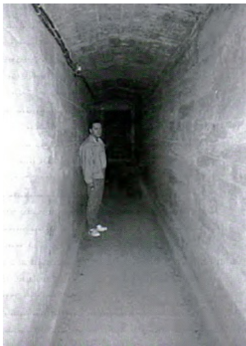
A Wartime Tunnel Beneath Fürstenstein Castle
