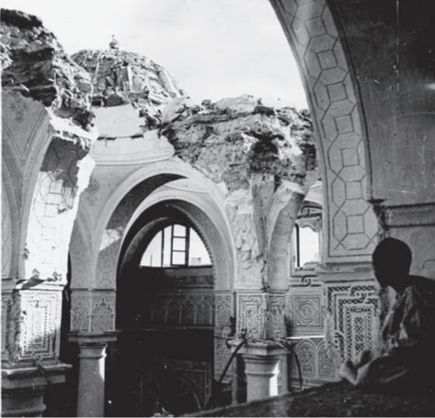
3.11 A destroyed mosque in North Africa, 1942 (BPK).
