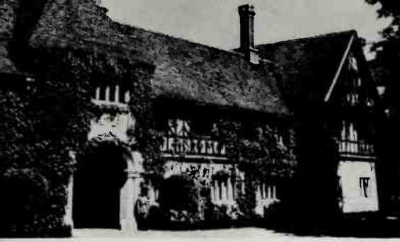
The conference building in Potsdam.
