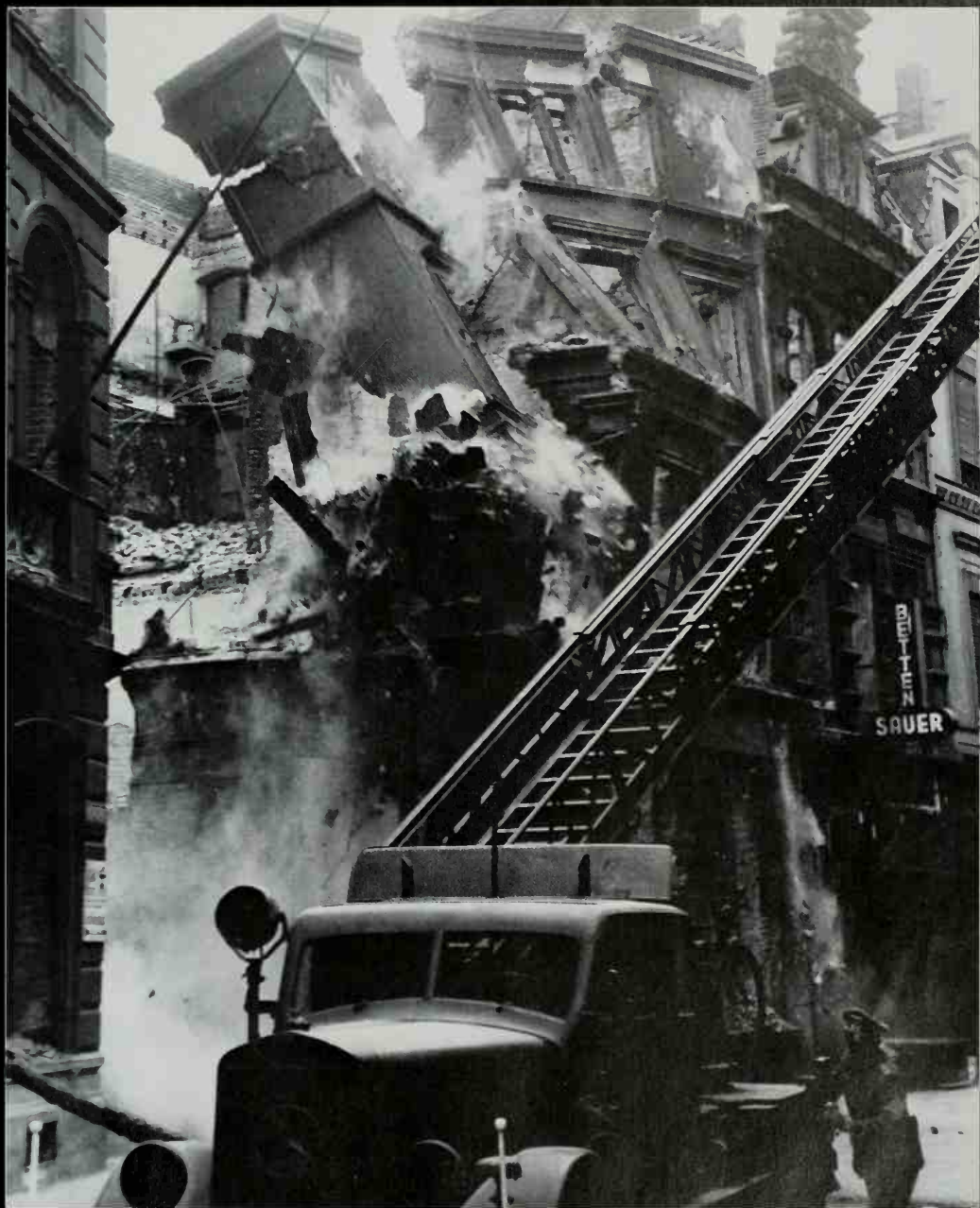
With the aid of a fire ladder and heavy cable, Wehrmacht soldiers demolish a gutted Cologne building, smashing its walls inward to spare passersby.
