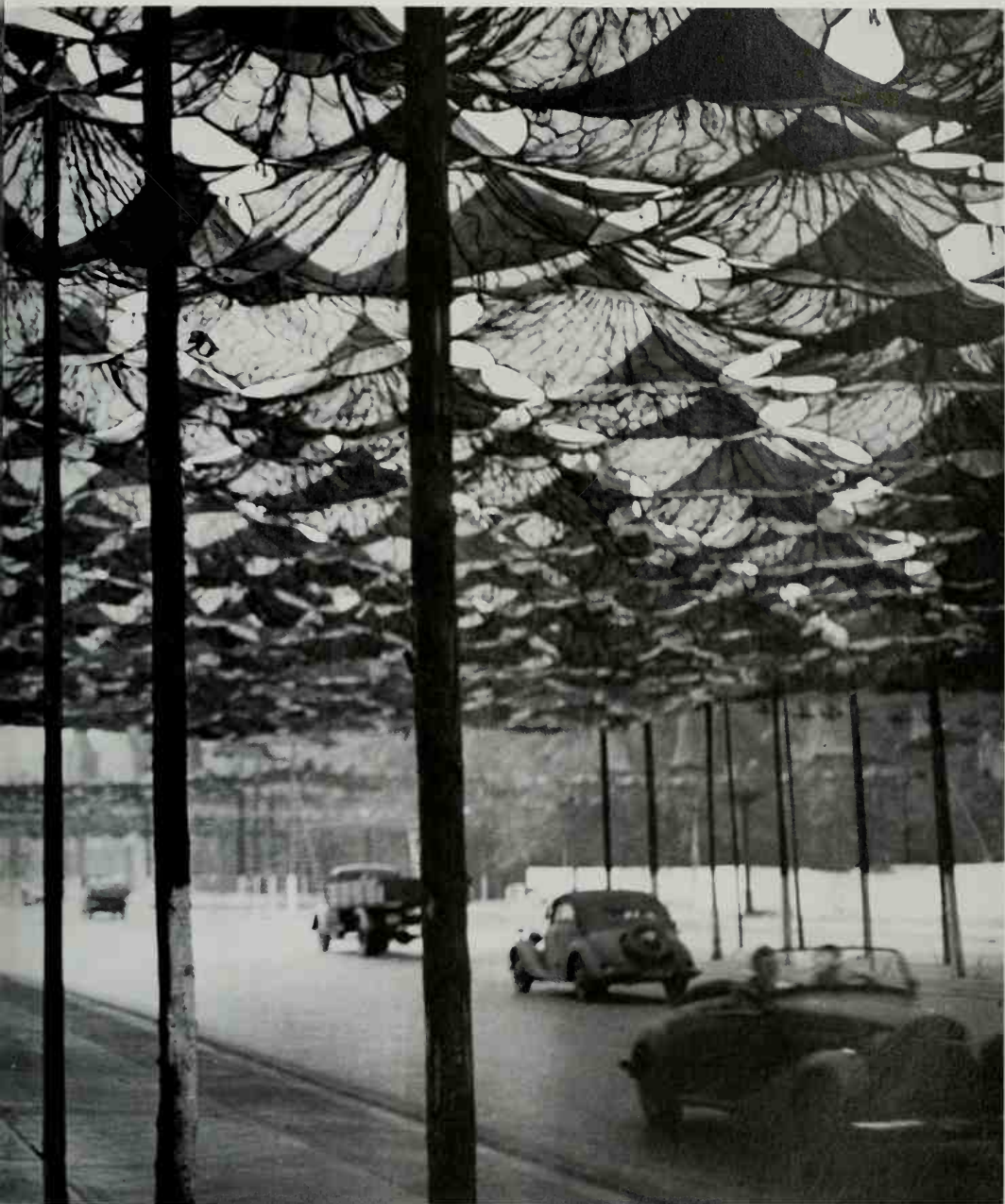
Berlin's Brandenburg Gate in late 1939. Strips of brown and green burlap laced in the netting simulated the evergreen groves that flanked the boulevard
