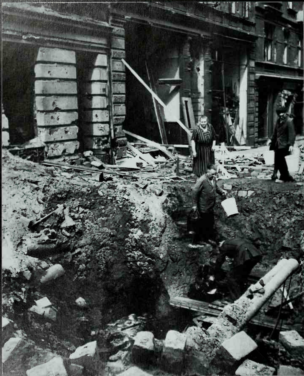
Hamburg citizens draw water from a picture frame. About 100 such watering holes had to be improvised after bombs destroyed 1,475 feet of water pipes.
