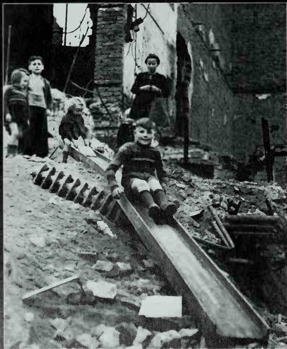
Children make a playground slide out of a twisted I-beam cast on a rubble heap.
