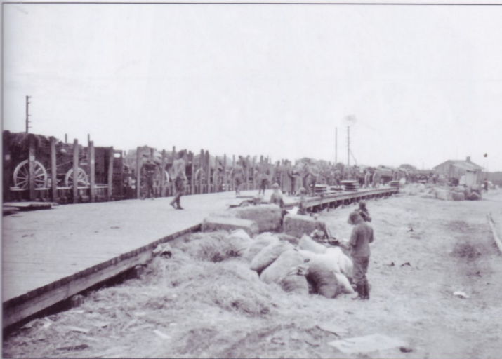
A wide-gauge railroad loading platform. These were built level with flatcars so that when they pulled in, there was a small gap between them and the platform, allowing loads to be entrained or detrained quickly and easily. The ever-present sacks of horse fodder and bales of hay can be seen stacked beside the platform.
