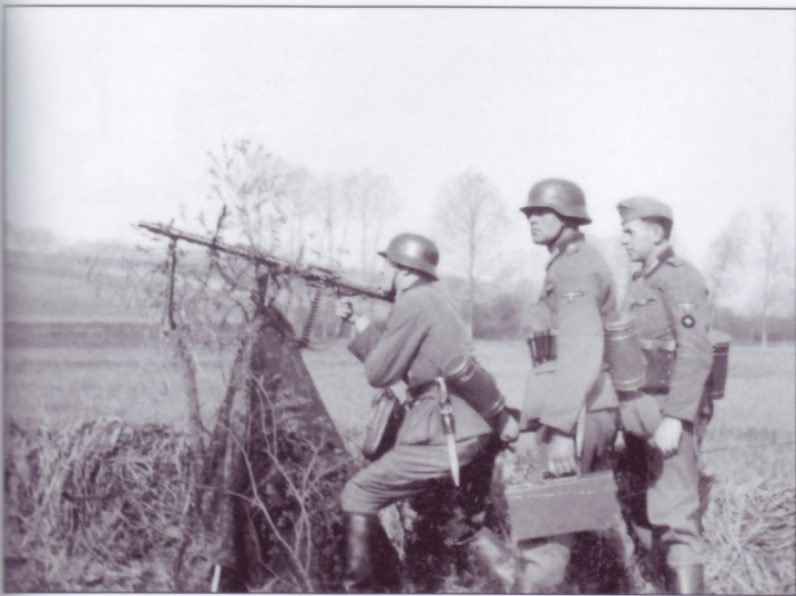
An MG34 machine-gun set up on an anti-aircraft tripod. The assistant gunner stands by with an M41 machine-gun ammunition box, which held either five 50-round belts (250 rounds, total) or a single 300-round belt. The first photo very clearly shows the shoulder-sleeve insignia, including the Waffen-SS eagle.
