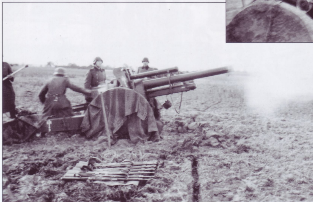
The photograph is blurred by the concussion of the gun firing as the lanyard is pulled. The Waffen-SS-pattern shelter-quarter covering the wheel is apparent. The gun tube of a 10.5cm le.FH18 had a life of 10,000 to 12,000 rounds before it had to be replaced.
