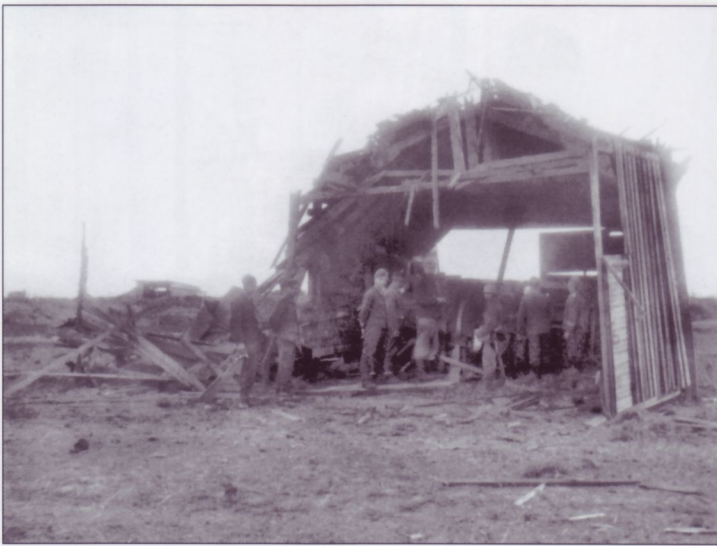
This hastily-built shelter was constructed from a destroyed barn. Like the previously-depicted log-framed shelter, it protected the gun, ammunition, and crew from the weather. Note the second shelter to the left on the skyline.
