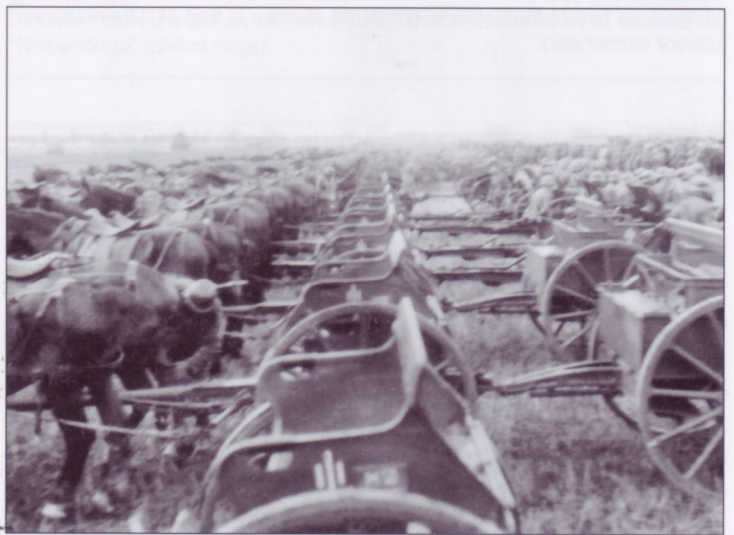
Another view of the same unit's light artillery limbers and caissons. Besides serving as limbers for artillery pieces they also towed ammunition caissons. The white artillery unit tactical symbol on the caisson's sides normally had the battery number (1 to 9) beneath it.
