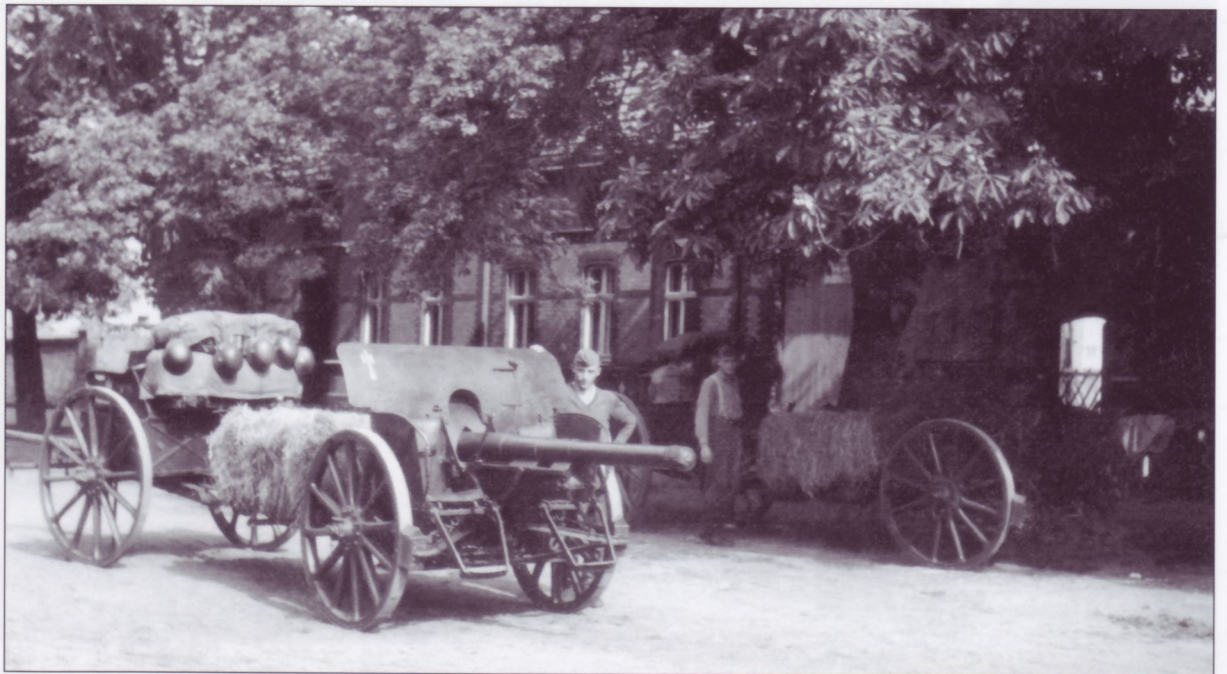
Another view of the same unit's light artillery limbers and caissons. Besides serving as limbers for artillery pieces they also towed ammunition caissons. The white artillery unit tactical symbol on the caisson's sides normally had the battery number (1 to 9) beneath it.
