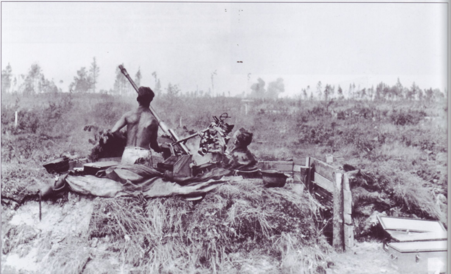
A 2cm FlaK30 crew fires on a Soviet aircraft. The earth parapet is reinforced with planks. This type of position was called a "Verstärkter Feldmässiger Ausbau", which was a deliberately constructed position of planks and timber, brick, or concrete. Such positions usually had a canvas tarp to cover the gun and its equipment. The number of guns assigned to light FlaK batteries varied over time, but was typically twelve 2cm and/or 3.7cm guns in four platoons of three.
