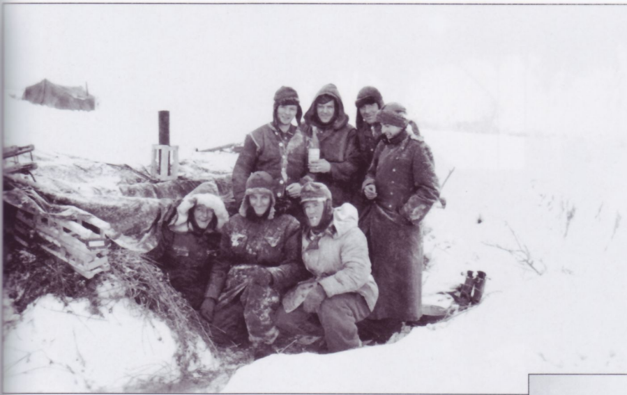
A gun crew poses before their hastily prepared dugout (Unterschleppe), or what soldiers called a dwelling bunker (Wohnbunker). Any and all materials were used to construct such shelters; artillery projectile packing frames have been used here. In the background is a large staff tent probably sheltering the Batterie - Trupp (battery headquarters).
