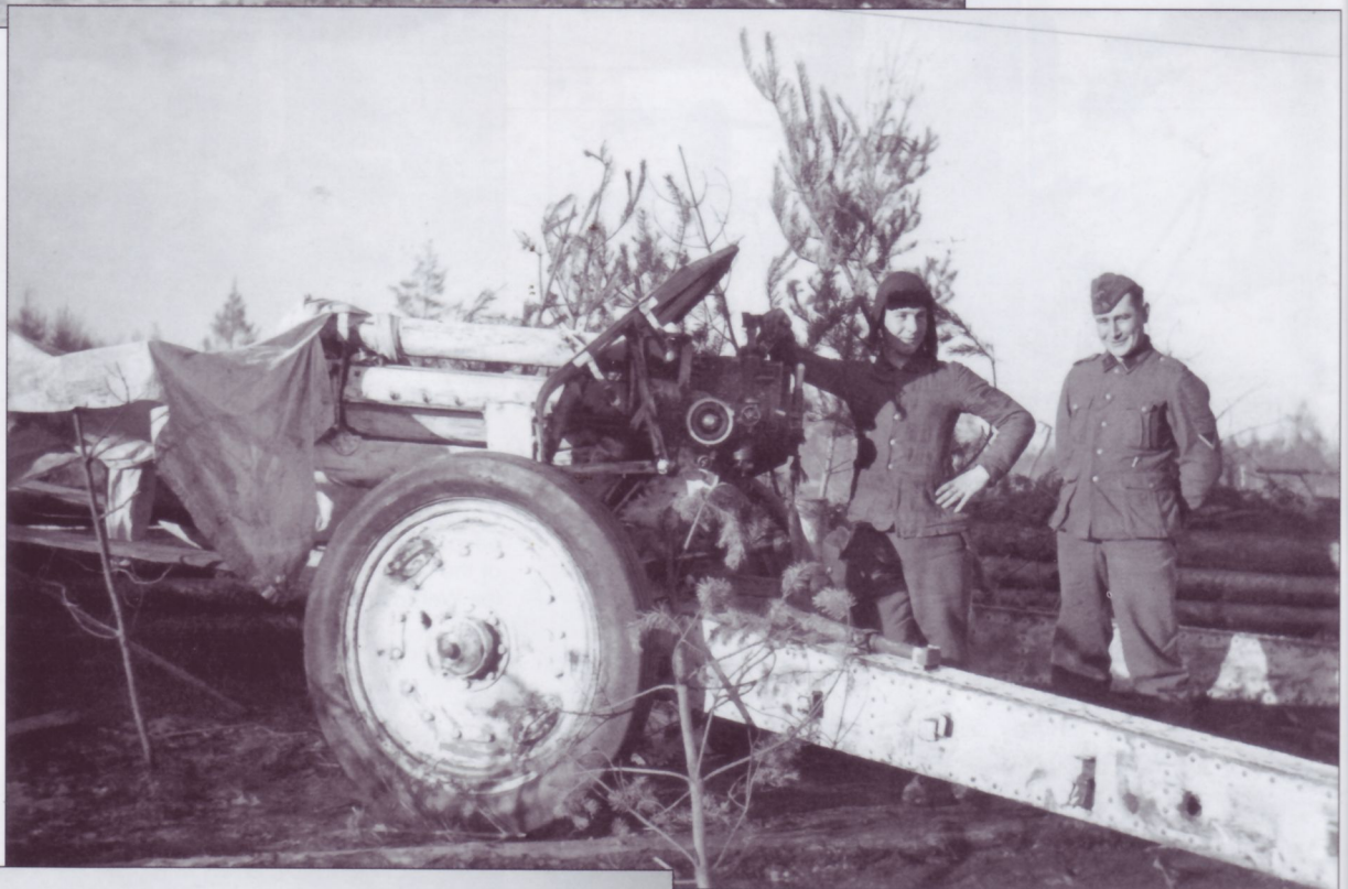
It was common for captured artillery pieces to be pressed into German service to make up for losses or augment the guns on hand. Here a Soviet 76.2mm M1927 infantry gun is limbered up. Four horses were required to tow the gun and its limber. It was typical for more gear to be carried on the limber, including personal baggage and spare clothing wrapped in canvas tarps. The Germans designated this piece as the "7.62cm Infanteriekanonenhaubitze (I.K.H.—infantry cannon howitzer) 290(r). In the center of this photo stands a Stabsgefreiter; the Waffen-SS eagle can be seen over his two rank chevrons. Heer rank insignia and Ordnungspolizei double-collar bars were still being worn at this time. The man to the right carries a collapsible canvas water bucket for the horses.
