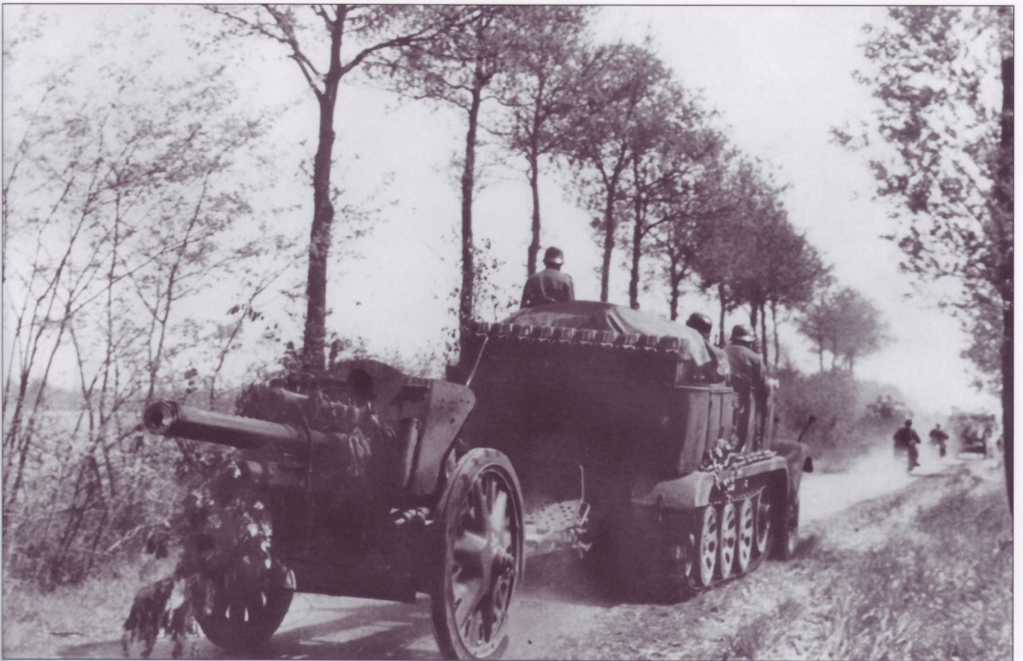
A mittlerer Zugkraftwagen 5-ton Sd.Kfz.6 halftrack prime mover tows a 10.5cm I.FH18 light field howitzer. This was the standard divisional artillery piece of both the Waffen-SS and Army.
