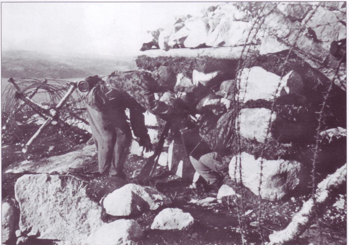
A hastily camouflaged forward command post or artillery observation post (often the two were combined), autumn 1943. Two camouflaged 6x30 Sf14Z scissors periscopes (Scherenfernrohr) can be seen in the position. Assorted equipment is strewn about in the foreground.
