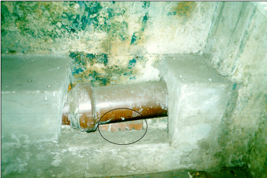
Photo 8: Delousing chamber in Stutthof, interior, west wall; cast iron connection pipe to the oven installed outside the gas chamber, which was used to heat the air. The pipe was originally surrounded by masonry, similar to that visible in the photo, but perforated. One of the perforated bricks is still visible below the pipe (circle). © Carlo Mattogno
