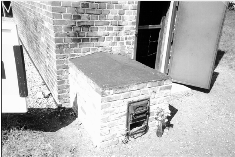
Photo 5: Delousing chamber at Stutthof, viewed from the south. The oven was used to heat the air inside the delousing chamber. © Carlo Mattogno
