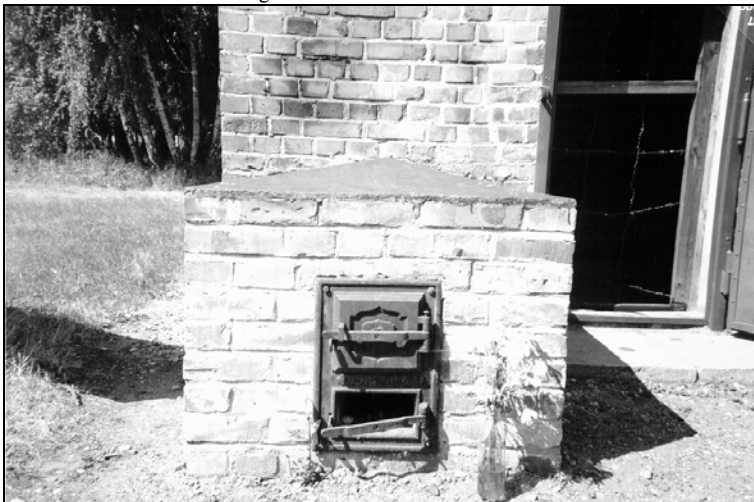
Photo 6: Delousing chamber at Stutthof, viewed from the south. The oven was used to heat the air inside the delousing chamber. Above: the fire door. Below: the ash door. © Carlo Mattogno
