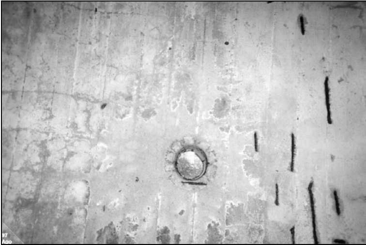
Photo 10: Delousing chamber at Stutthof, interior. Circular opening in the middle of the reinforced concrete roof. Note the typical blue pigmentation caused by iron cyanide. This opening was used for the introduction of Zyklon B into the delousing chamber. © Carlo Mattogno
