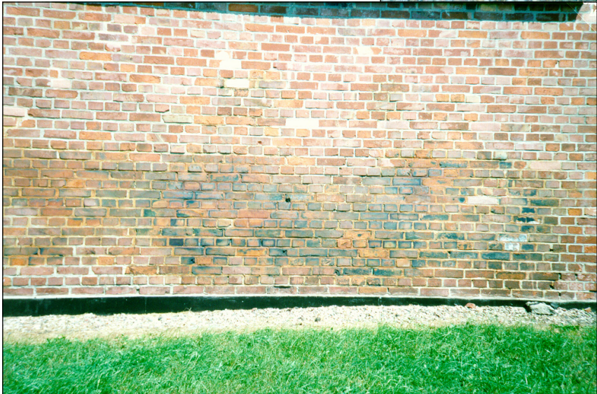
Photo 17: Delousing chamber in Stutthof, east side. Blue stains on the wall are proof of the use of Zyklon B. © Carlo Mattogno
