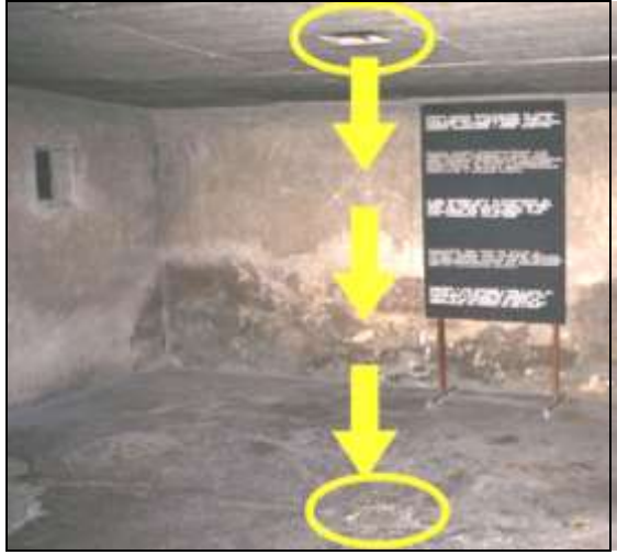
Figure 10: Morgue in the New Crematorium of the Majdanek camp, prior to museum revisions. A crudely cut hole in the ceiling was for decades alleged to have been used to drop Zyklon B pellets into the room to gas trapped victims – although those pellets would have fallen directly into a floor drain below. This sign, now removed and revised, deceitfully claimed this was a homicidal gas chamber.
