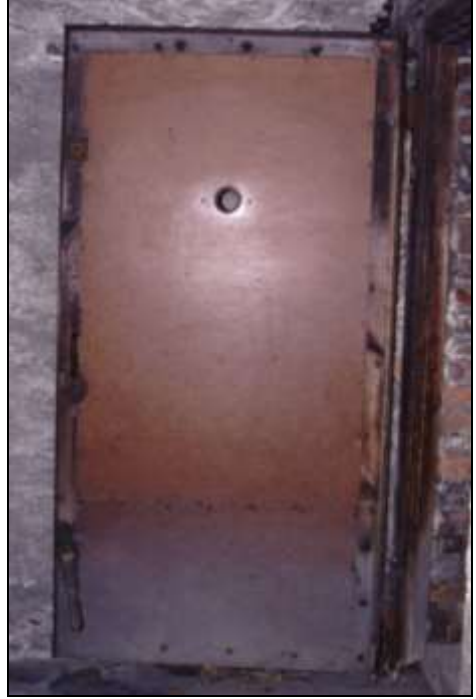
Figure 23: Makeshift air-raid-shelter door of Krematorium I made of wood with a thin sheet-metal cover, probably built by inmates in the camp's workshop.
