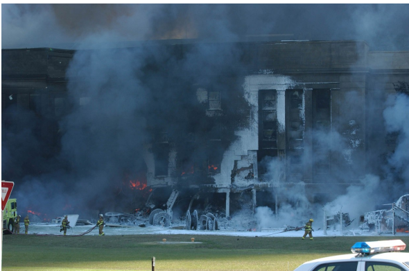
Notice the roof line of the building is still in tact with unbroken windows
