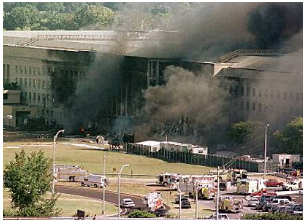
Roof line still intact with no visual crash debris present
