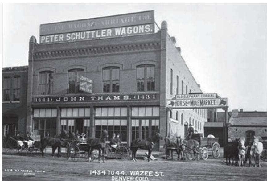
John Thams building and entrance to the Elephant Corral, ca. 1900. Courtesy, Denver Public Library.
