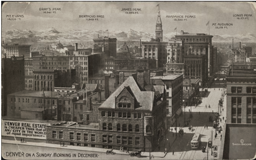
The original Denver Club building, which opened in 1889, sits in the foreground of the Denver landscape near the turn of the century. Courtesy, History Colorado, Denver.
