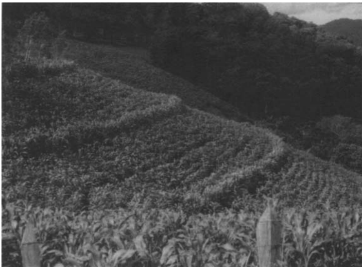
PHOTO 8.1. A hillside showing contour ditch-bund structures designed to slow and capture flowing water.
