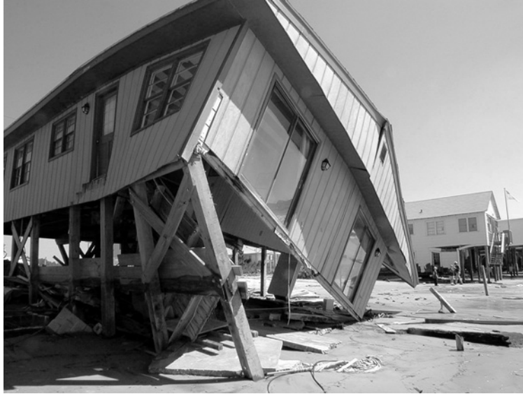
FIGURE 5–2 South-facing Long Beach on Oak Island, North Carolina, September 17, 1999. Hurricane Floyd brought a devastating 15 feet of storm surge that damaged or destroyed hundreds of houses along this community's oceanfront and flattened its frontal sand dunes. Here, even elevation failed to save this home. Additional strapping, upgraded mitigation work, might have helped. Photo by Dave Gatley/FEMA News Photo.
