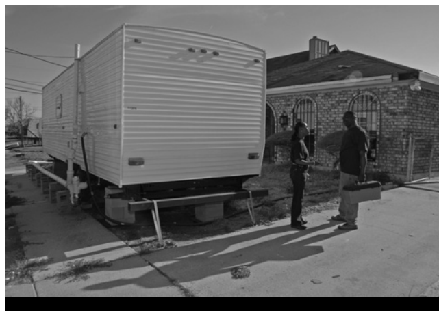
New Orleans, LA, March 7, 2006 On day 2 of moving in, Dionne Roberts stands by her FEMA trailer giving instructions to her plumber Glen Harris about repairing leaking water pipes in her house. Marvin Nauman/FEMA
