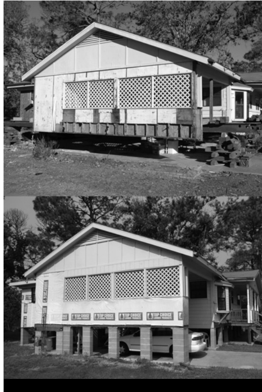
Pascagoula, MS, November 29, 2005 and August 8, 2006 Before (top) and after the elevation of a house flooded by the storm surge of Hurricane Katrina. Elevating a house is an excellent method to mitigate against flooding.
