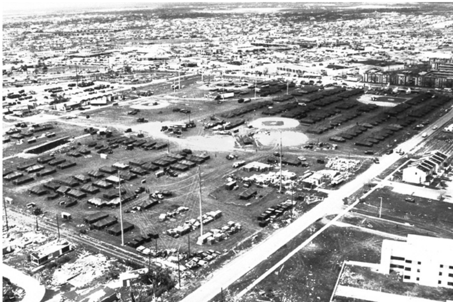
FIGURE 2–3 Hurricane Andrew, Florida, August 24, 1992. An aerial view showing damage from one of the most destructive hurricanes in America's history. One million people were evacuated and 54 died in this hurricane. FEMA News Photo.
