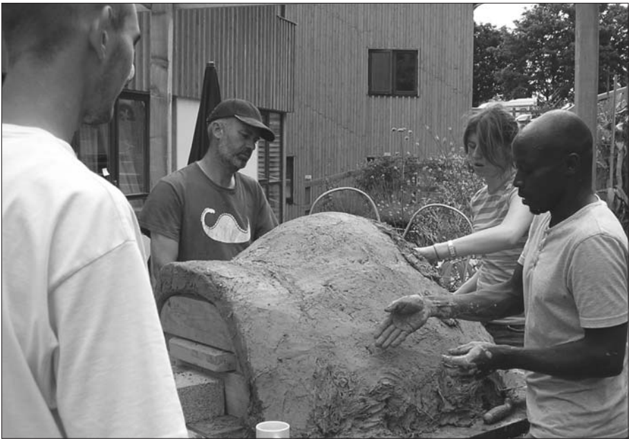
Photo 6.1 Conviviality: Building the bread oven at Springhill co-housing, June 2008
