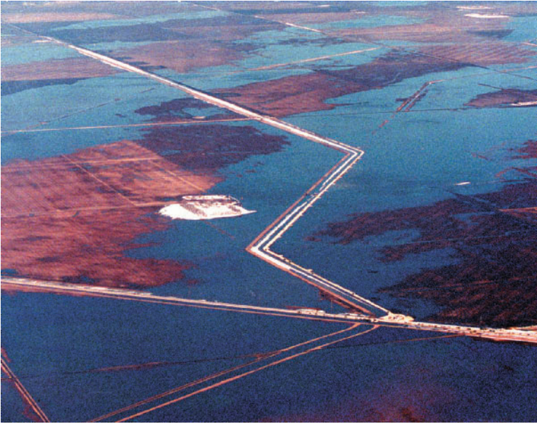
PLATE 6 The 15-mile Brunkild Z-dike was constructed out of mud, sand, and limestone in 72 hours (courtesy of Winnipeg Free Press).
