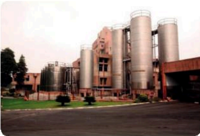
▲ The Amul plant in India showing the milk silos
