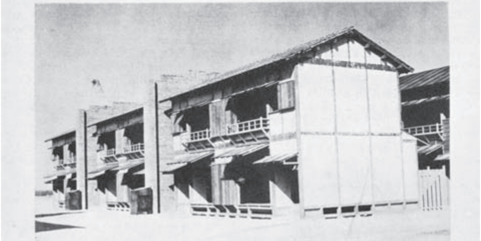
Views of German and Japanese residences in the 1943 incendiary bomb test villages at Dugway Proving Ground, Utah. Chemical Warfare Service/National Defense Research Committee
