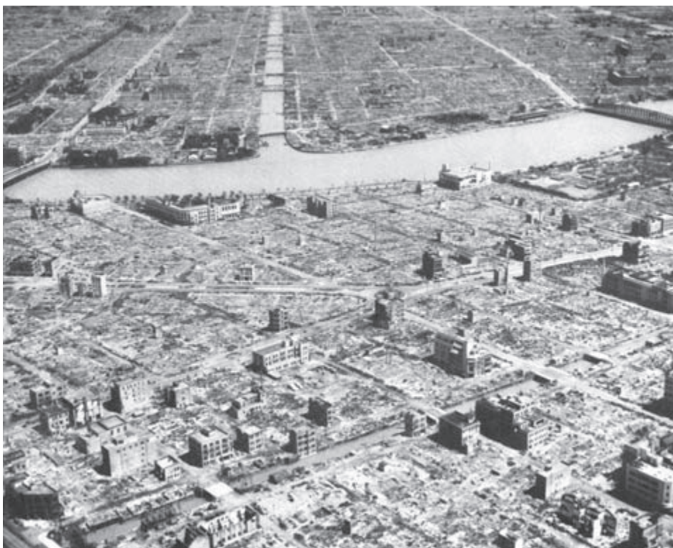
Tokyo's Nihonbashi District after attacks with napalm and explosives. Concrete buildings are gutted. All other structures have been obliterated. U.S. Army
