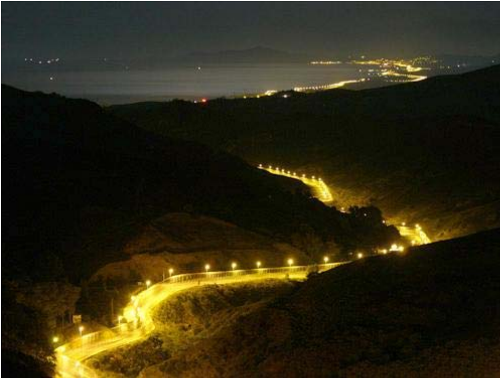
Ceuta border fence between Spain and Morocco
