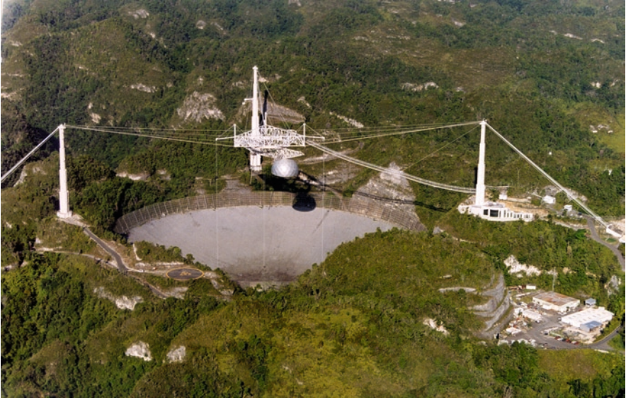
Fig. 5.3 Parabolic antenna of Arecibo's radio telescope, 305 m in diameter. The Gregorian dome is suspended from three gigantic columns, where signals collected by the principal antenna are detected. At the right , note the building complex at Arecibo's Observatory. Courtesy of Daniel R. Altschuler/Arecibo Observatory
