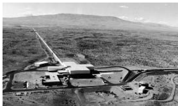
FIGURE 30 LIGO, in Washington State, consists of two 4-km arms at right angles, each with laser beams in high vacuum. There is an identical observatory in Louisiana, and the two installations will work in tandem. The objective will be to detect gravity waves by searching for changes in length a thousand times smaller than an atomic nucleus.
