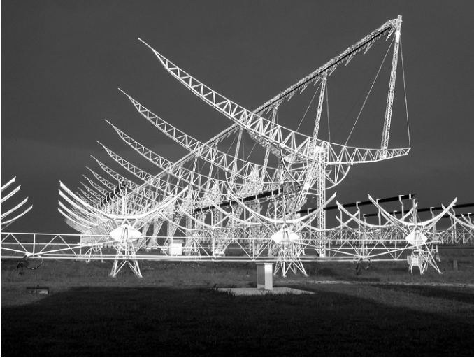
Figure 15.3 The large T-shaped Northern Cross Array, 560 meters (East-West arm) \times 640 meters (North-South arm) composed of some 5632 dipoles.
