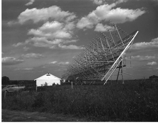
Figure 4.1 The first radio telescope designed and constructed by John Kraus.
