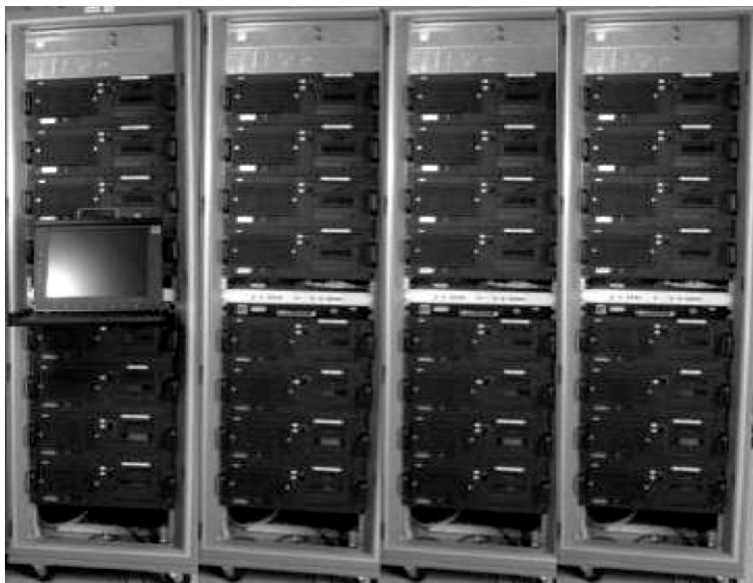
Figure 9.5 Prelude system hardware based on rack-mounted PCs, each with two custom accelerator cards.
