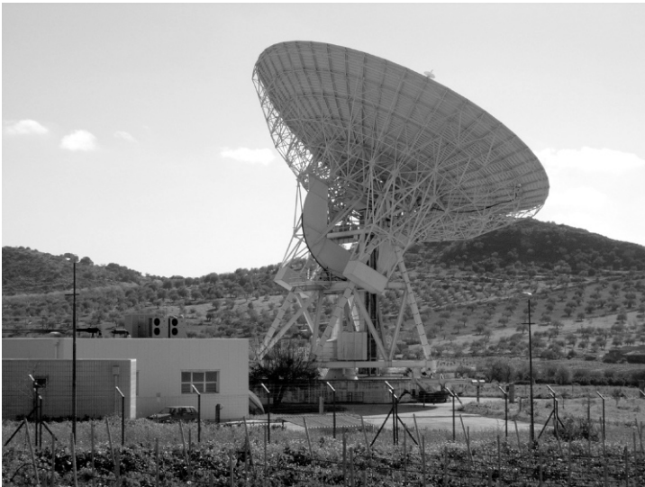
Figure 15.2 The Noto 32-m VLBI dish, equipped with an active mirror that allows it to operate at F_{\max} > 33 GHz.
