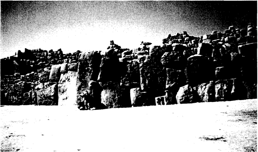
The massive walls of Sacsayhuaman, above Cuzco.
