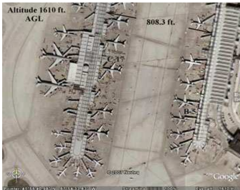
Figure 1. Aerial Photograph of United Concourses B and C from Altitude of 1,610 Feet.
