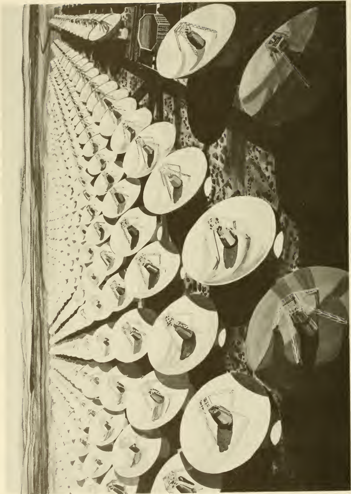
View 3. Artist's concept of low aerial view of the Cyclops system antenna array, showing the central control and processing building.
