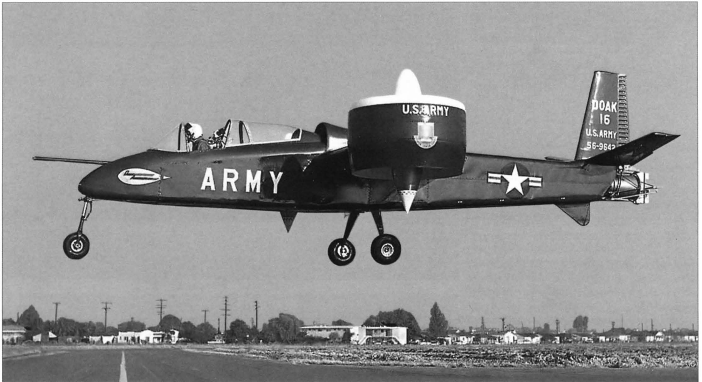
The Doak Model 16 experimental VTOL aircraft flown by Jim Reichert makes a test flight in 1958 at Torrance Airport, California. Doak Aviation
