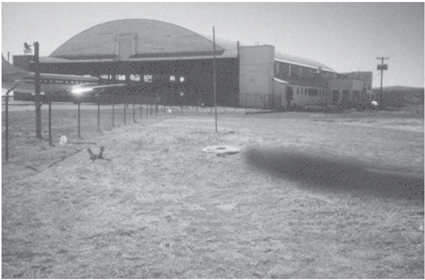
Hangar P-3 today (Building 84).
