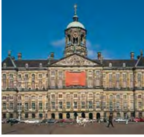
مبنى البلدية mabna al-baladeeya town hall
