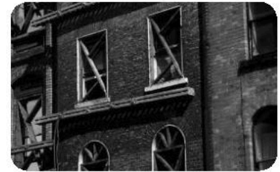
A house near a bomb site
