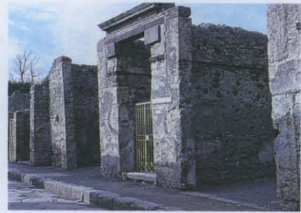
The front of Caecilius' house. The spaces on either side of the door were shops he probably owned.
