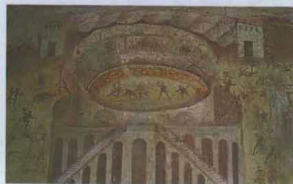
Bird's-eye view of the amphitheatre showing the awning.
