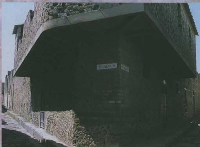
A house with its first storey overhanging the road to gain a little extra floor space; often the first floor was a separate flat. (The street signs are modern.)
