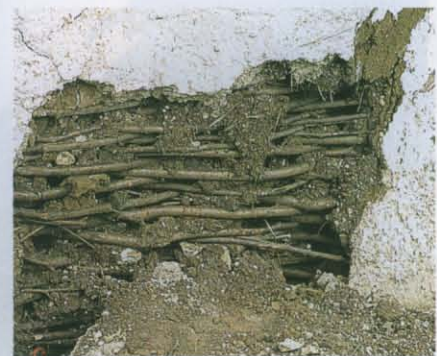
Wattle and daub: basketwork covered with clay.
