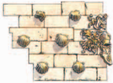
STONE WALL, QUOINS, AND SHELL DECORATION, CASA DE LAS CONCHAS, SALAMANCA, SPAIN, 1475-1483
