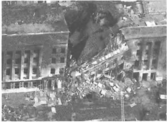
Figure 48: This is the image that people remember of the collapsed wall of the Pentagon, but this didn't happen until half an hour or more after 'impact'. Before that time the hole was tiny compared with the size of a 757.
