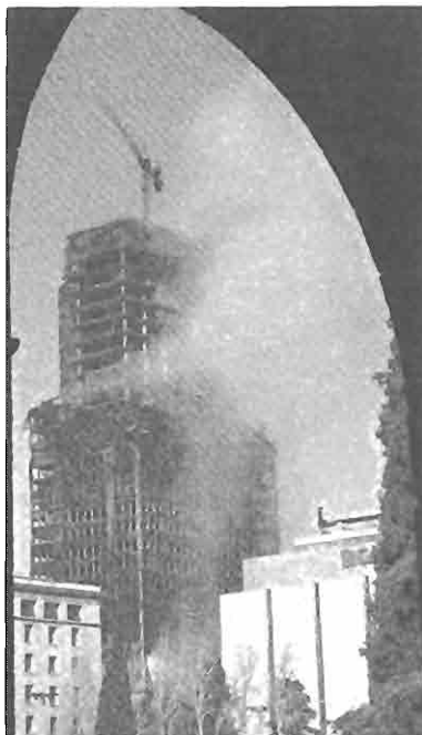
Figure 63: The steel-framed high-rise Windsor Building in Madrid burned with far greater intensity than the Twin Towers in 2005 and for far longer – the fire took 24 hours to extinguish. It did not collapse.
