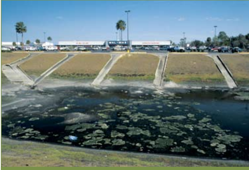
Polluted runoff from a shopping center parking lot in Inverness, Florida, is stored in a drainage pond. (© Jeff Greenberg / The Image Works)
