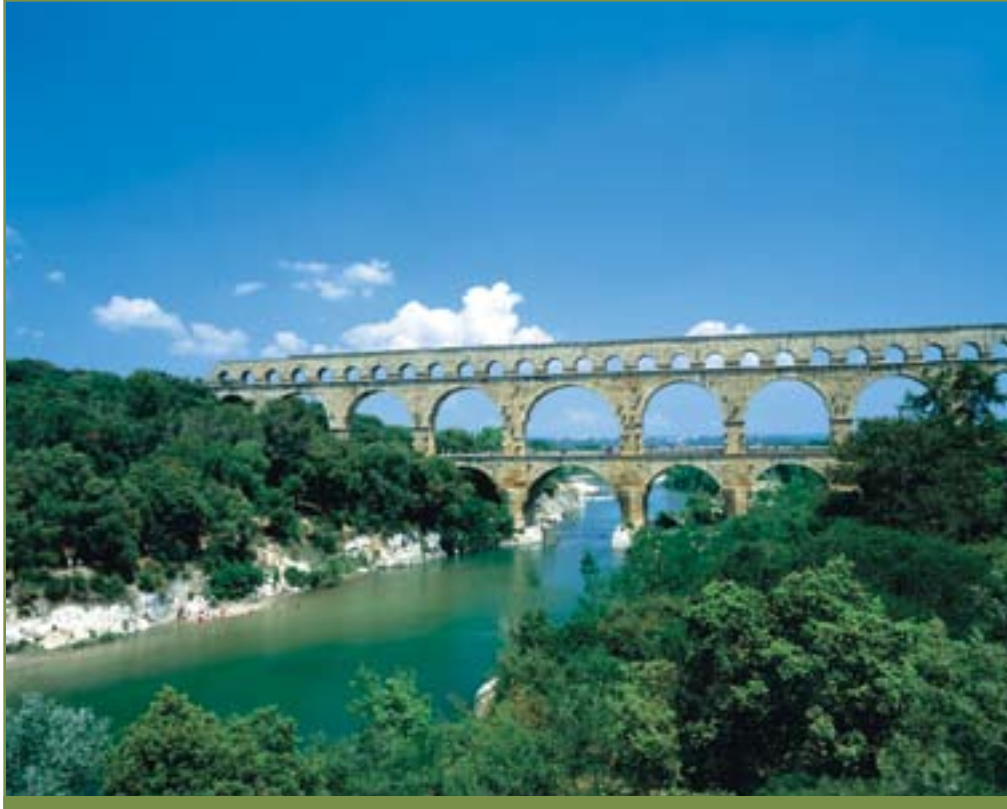
The incredibly well-preserved aqueduct at Pont du Gard, Provence, France, illustrates how the Romans transported water to their settlements. ( © age fotostock / SuperStock )
