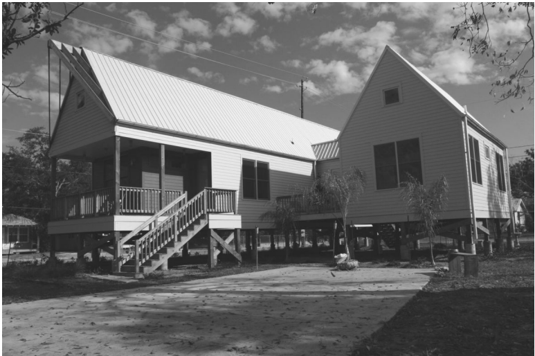
Figure 13.1 The Parker Residence, designed by Brett Zamore Architects to house a family of six, cost $130,000 to build in 2007. AFH’s Biloxi Model Home Program facilitated its funding, design, and construction. Photograph by Alan Richardson, provided by Architecture for Humanity under Creative Commons licensing.
