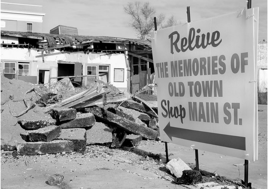
Bay St. Louis businesses have been besieged by years of constant construction, their woes compounded by astronomical insurance rates.
