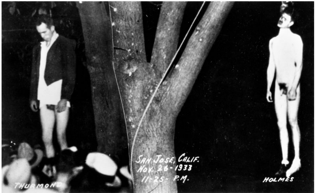
FIGURE 6.11 The lynching of Thomas Thurmond and John Holmes, San Jose, California, 1933. This postcard was constructed from two photographs of the men. Prints and Photograph Division, Library of Congress, Washington, D.C. Courtesy of the National Association for the Advancement of Colored People.
