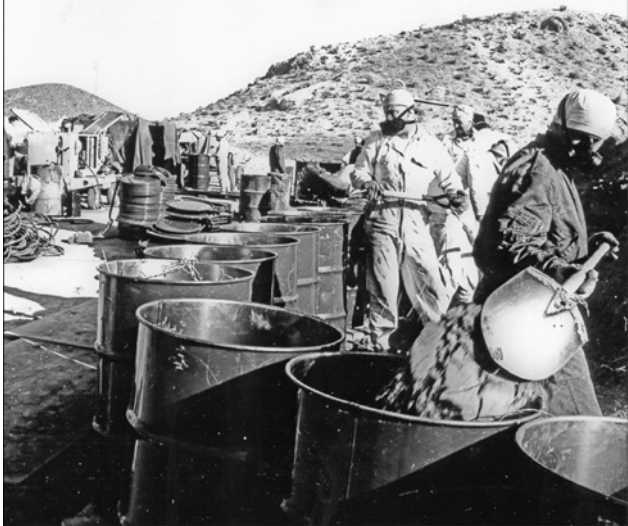
The most contaminated dirt was packed into 4,810 barrels for shipment to the Savannah River nuclear processing center in South Carolina. Courtesy of Sandia National Laboratories
