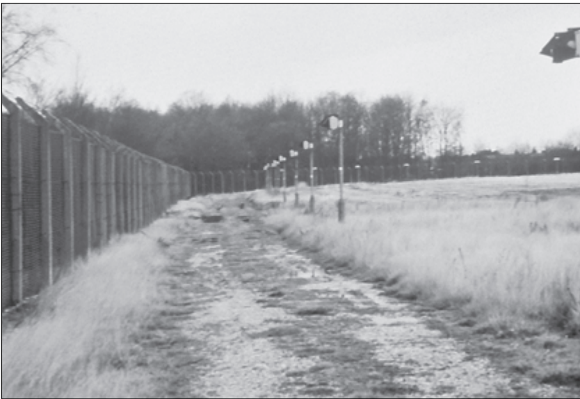
Figure 8.10. The perimeter fence in situ with an internal road and security lighting. © West Berkshire Heritage Service 2868
