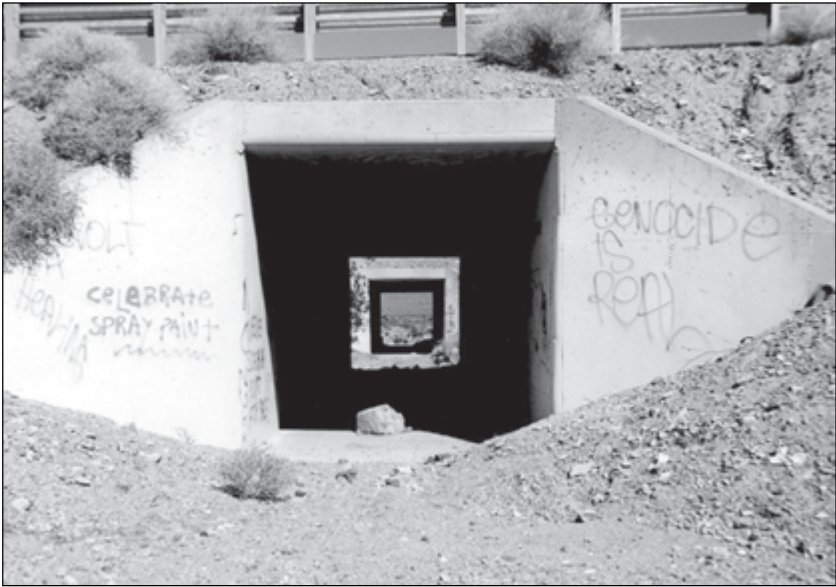
Figure 17.13. Tunnels under the highway.
