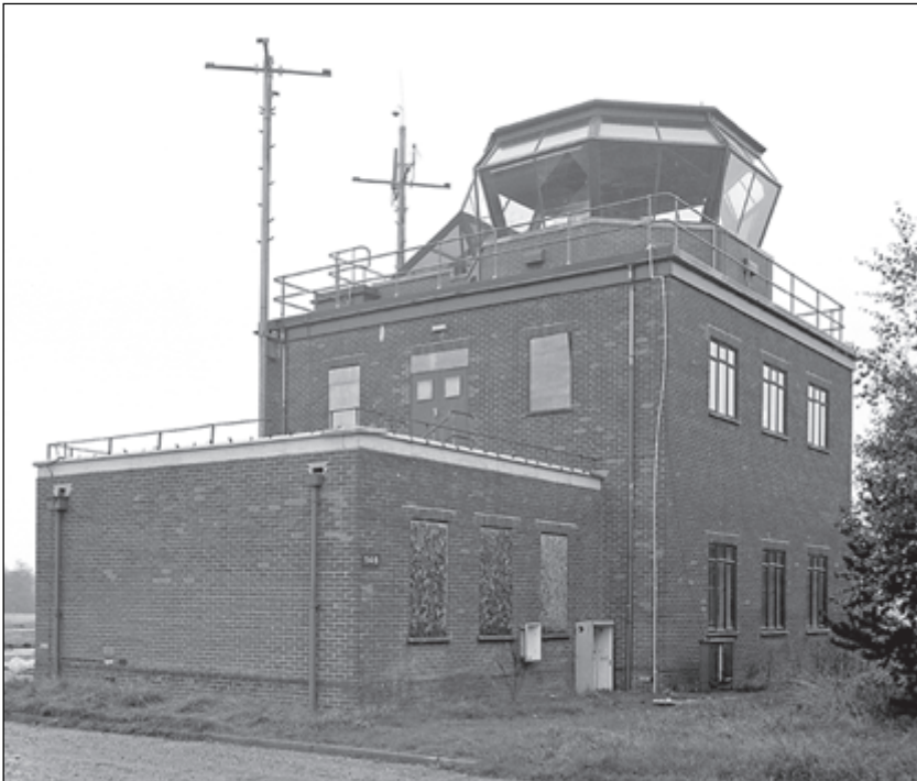
Figure 8.13. The Control Tower (a USAF type 5222A/51 tower) dates to the early 1950s and was built during alterations to the airfield to accommodate the USAF Strategic Air Command. The structure is currently secured for its protection until a long-term use can be determined. © English Heritage AA003331
