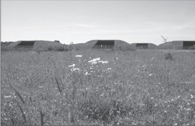
Figure 8.1. Greenham Common, West Berkshire: the iconic cruise missile shelters of the GAMA site contrast with the restored heath. © Veronica Fiorato
