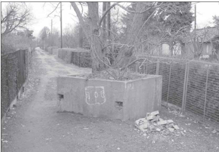
Figure 11.5. Flower bowl barricade made from a BT9 watchtower element. Photo by L Schmidt
