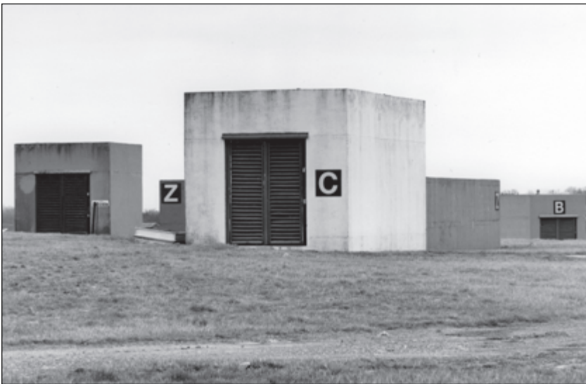
Figure 7.6. RAF Ash, Kent. A former radar station, this surreal landscape of lettered concrete ventilation cubes reveals little of the intense building activity that took place below ground during the 1980s. © Crown copyright NMR AA96/03084
