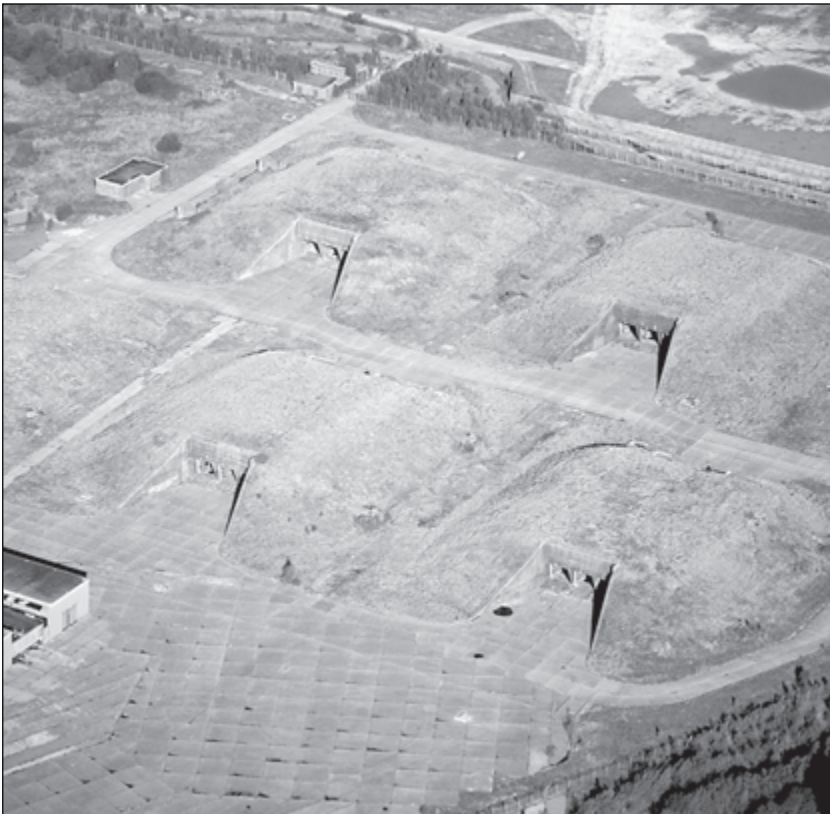
Figure 8.3. The GLCM Alert and Maintenance Area or 'GAMA'. The six cruise missile shelters are surrounded by a triple fence which also encloses ancillary buildings. These include a vehicle maintenance facility (bottom left), a fire team building and generator house (top left) and a guard house by the main entrance (top centre). One of the shelters (top centre) was manned 24 hours a day to provide an immediate response in an emergency. © English Heritage NMR 21863/13
