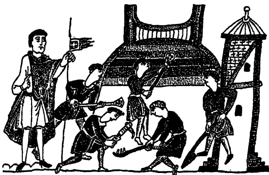
FIGURE 6.—CONSTRUCTION OF A CASTLE AT HASTINGS
