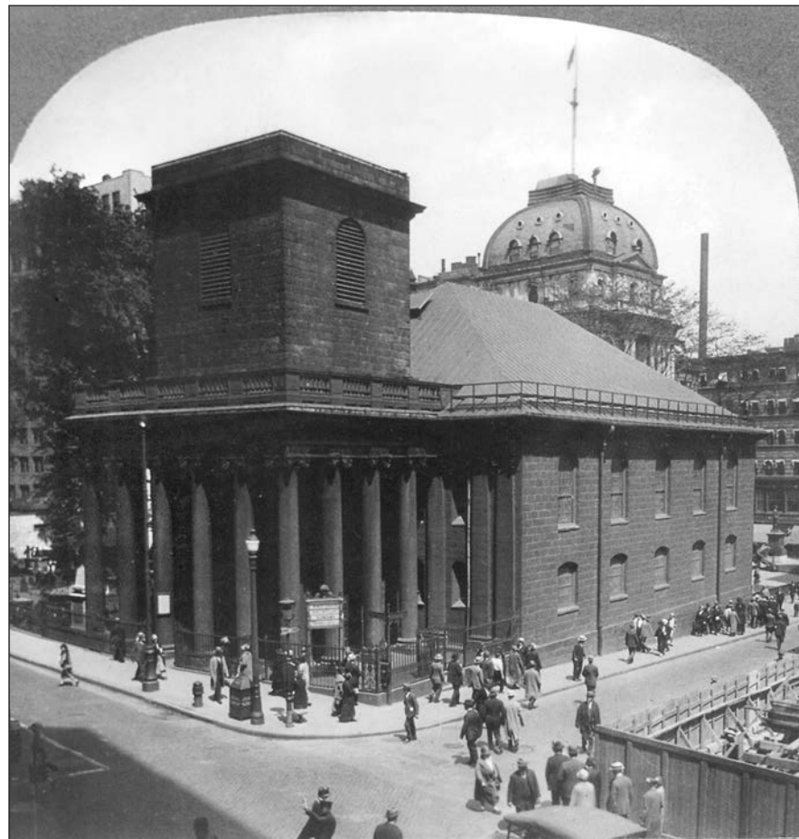
King's Chapel (built 1749–1750) in Boston is distinguished as the first American church constructed of stone. Rectangular in plan with a hipped roof, its interior has elegant classical details including Corinthian columns supporting the gallery.
