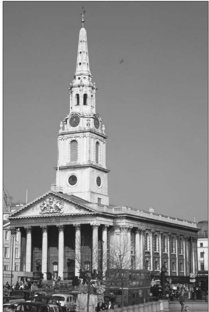
James Gibbs’s St. Martin-in-the-Fields Church (built 1722 to 1726) in London was the most influential and most frequently imitated church, particularly after the mid-eighteenth century.
