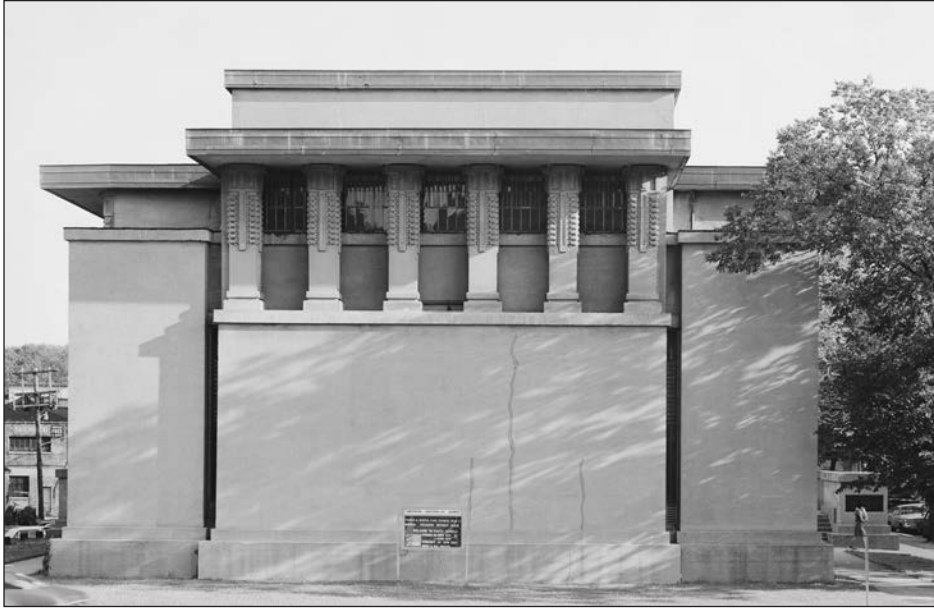
Frank Lloyd Wright's Unity Temple in Oak Park, Illinois (1906), among the first twentieth-century churches whose design did not reflect a stylistic precedent, was built of concrete in a square configuration.
